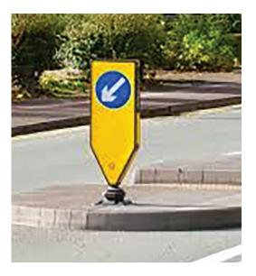
These raised medians are a safe place for pedestrians to wait before they finish crossing the road. By crossing in two stages, they can deal with one direction of traffic flow at a time.
